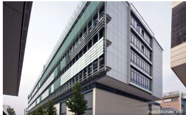
Fraunhofer-Institutes IPA & IGB, Stuttgart New unit D
