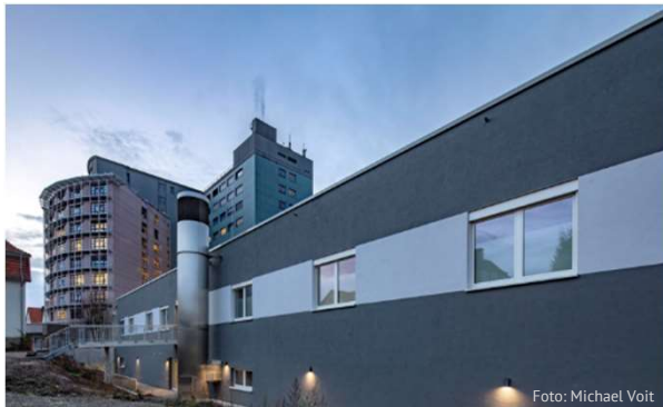
Clinic Werra-Meißner Hospital Eschwege New building, functional tract 1a
