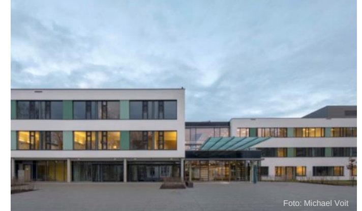
Konstanz Clinic New functional building and Vincentius Hospital
