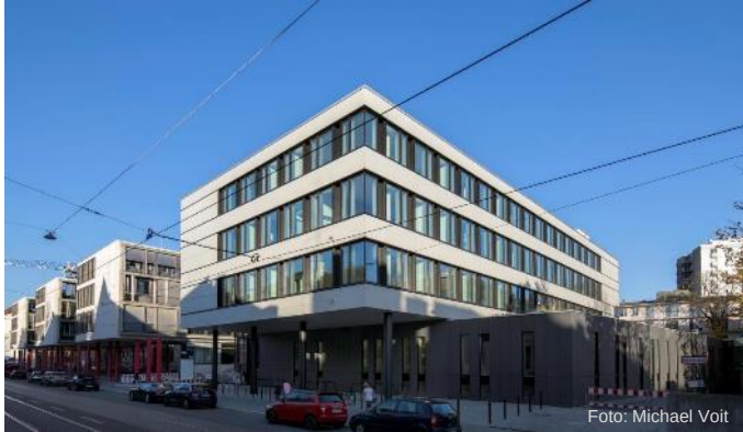
Clinic r. d. Isar, München New operation center north
