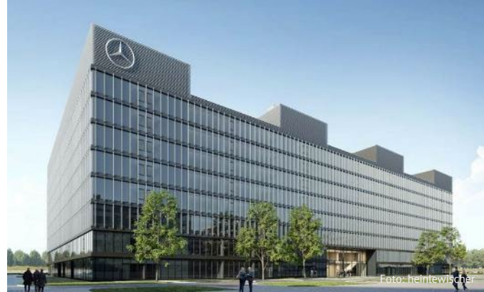
Daimler Sindelfingen New center for electric integration ESH with test bench, body shop and administration
