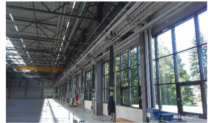
Viega, Plant Elspe New unit 13, industrial warehouse, administration
