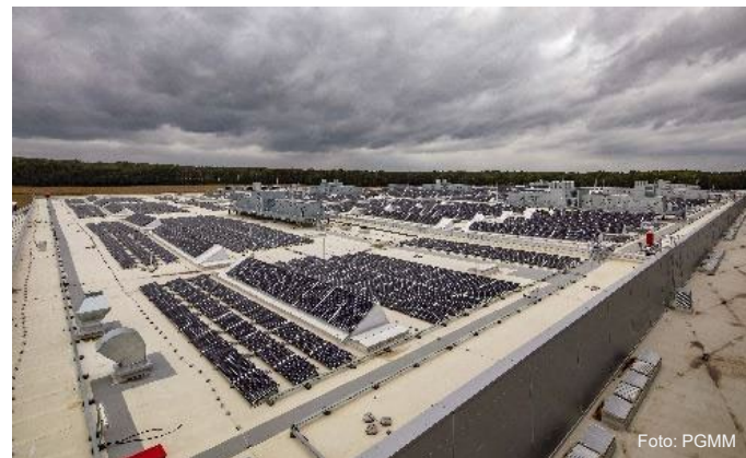
ACCUmotive Kamenz Expansion production site, Plant II
