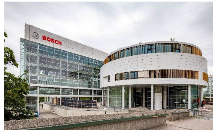
AER Fritz 9 München Reconstruction and Expansion
