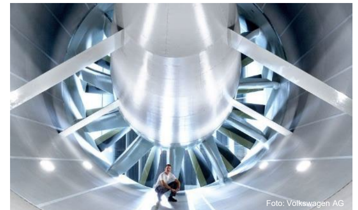
VW Wolfsburg, Center of efficiency for undergrate air duct
