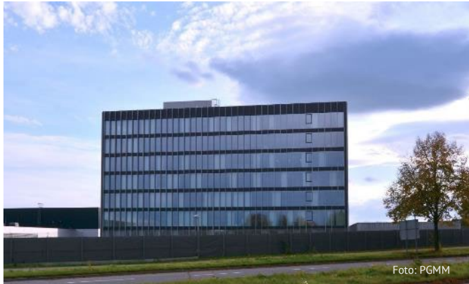
Daimler FLX Engineering Sindelfingen New administration building with energy canal Hse.64/5&EK847
