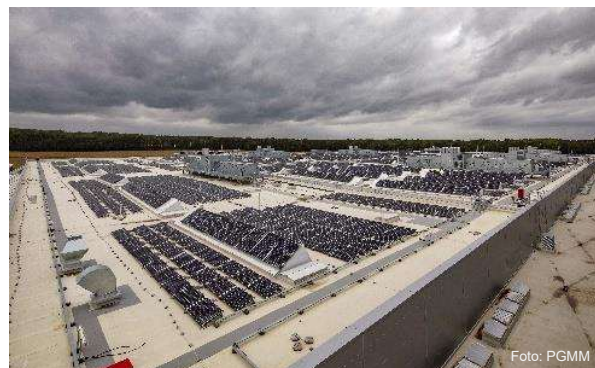
ACCUmotive Kamenz Expansion production site, Plant II
