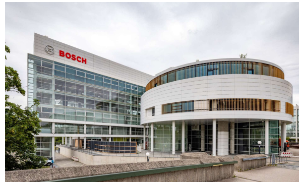
AER Fritz 9 München Reconstruction and Expansion
